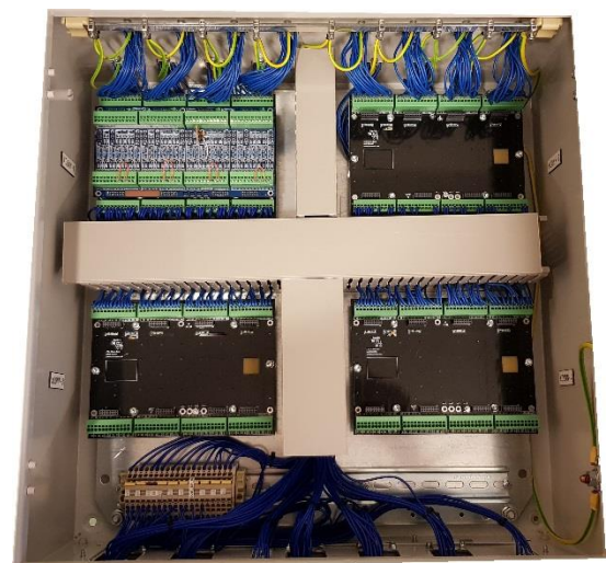
Picture: LP339 interior with one X-CONN-card.
